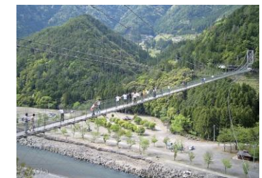
Suspension Bridge of Tanise (Nara)
